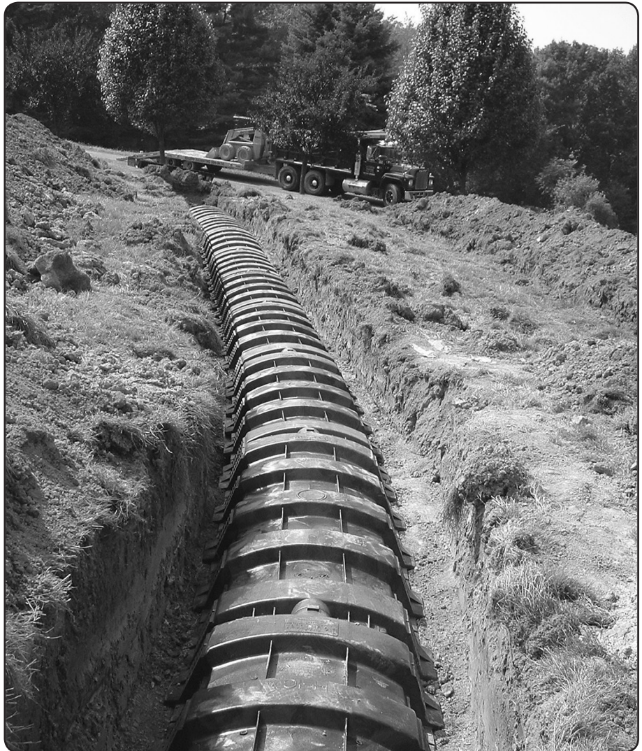
A layout of the second drainfield. □□
