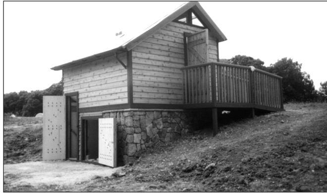
This restroom facility is located at Quail Ridge Park in St. Charles, Missouri. The basement holds two composting reactor tanks. Solar radiation provides both heat and electricity to the building. Photo courtesy of Kevin Mills.
