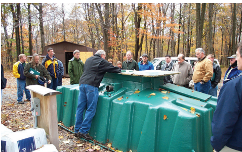
Peat filter module at the WV Onsite Demonstration Center
