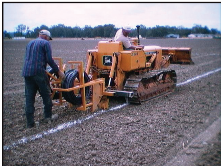
Figure 3: Typical installation of drip irrigation tubing Photo courtesy of GEOFLOW
