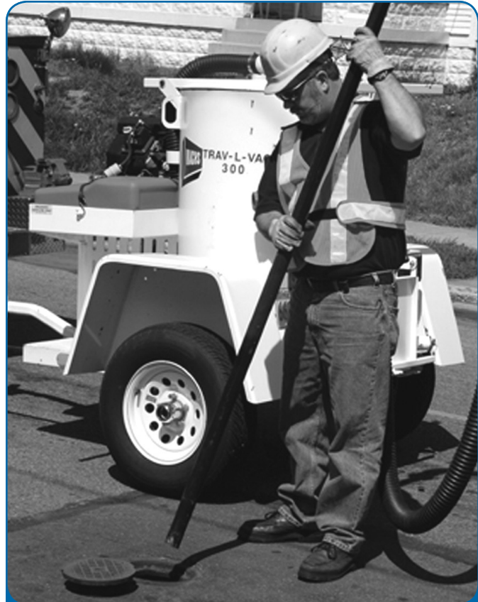
A worker cleans out the valve box with a utility vacuum cleaner. Removing accumulated sediment and dirt from the gate valve curb box must be done before exercising valves.
